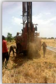
DRILLING AT HOSPITAL OF HOPE
